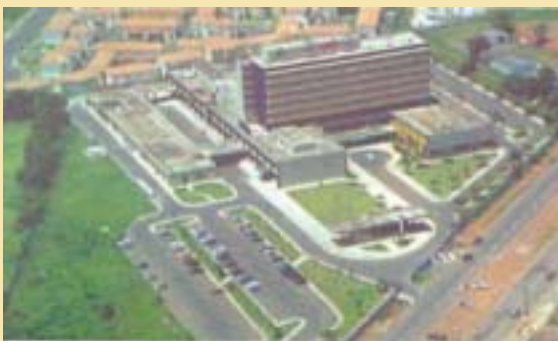
Hospital Estadual de Sumaré (SP)
